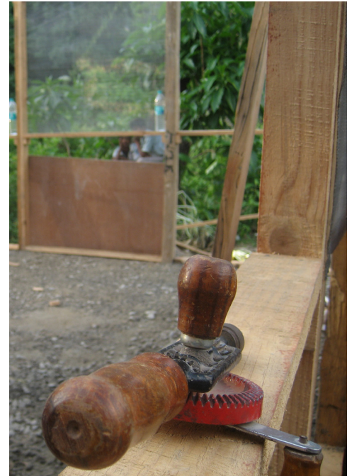
the hand-drill used for the construction of the shelter
