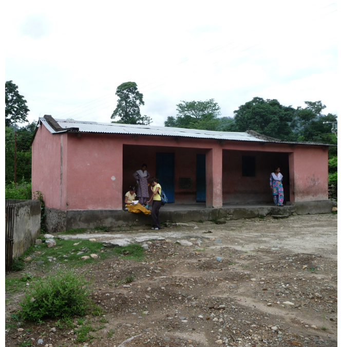
existing school building seen from across the yard
