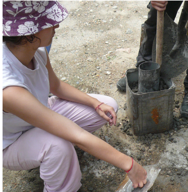
preparing the foundations
