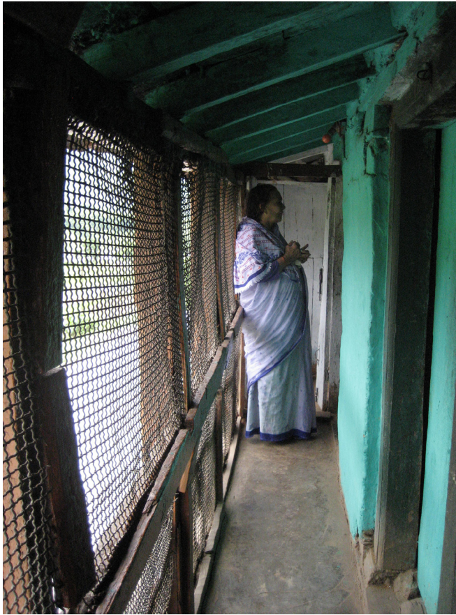
the balcony used for circulation
